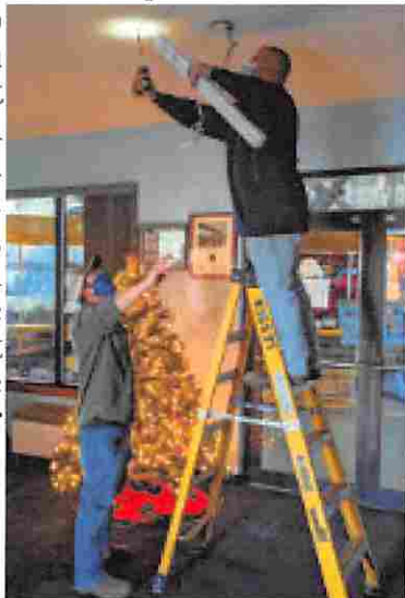
Electricians install our new lights
